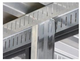
For Special Order Nonstandard Leg Lengths greater than 2.5" the slot length remains the same and is centered on the leg.
